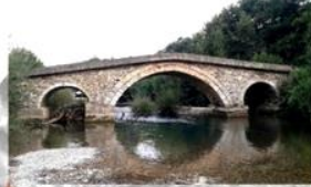
BRIDGE ON BISTRICA RIVER
