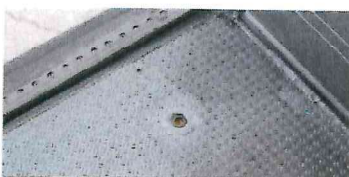
Drain in the floor pan.
